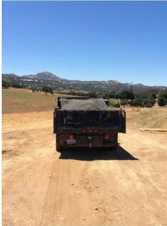
Photo 3: Spoils removed from Pole Z293923 (TL 625C) were covered in haul trucks to prevent fugitive dust in accordance with APM AIR-02.
